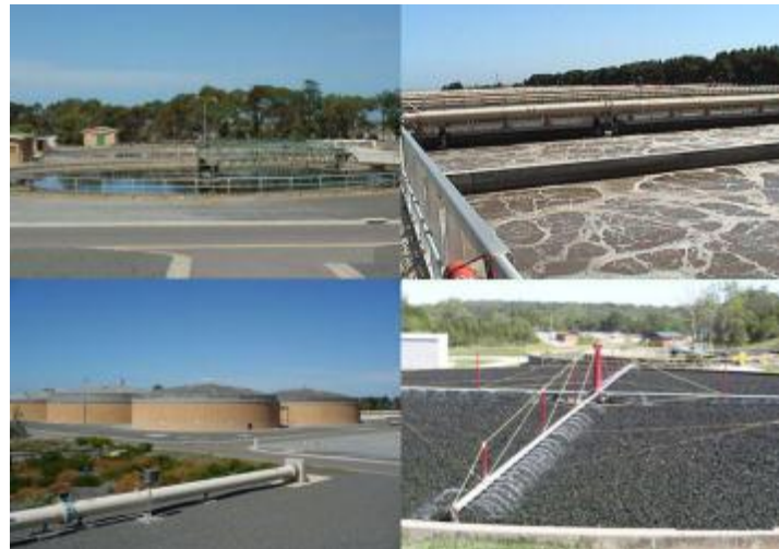
Common effluent treatment plant
