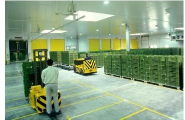
Hi-tech Cold Storage : 5000 MT
